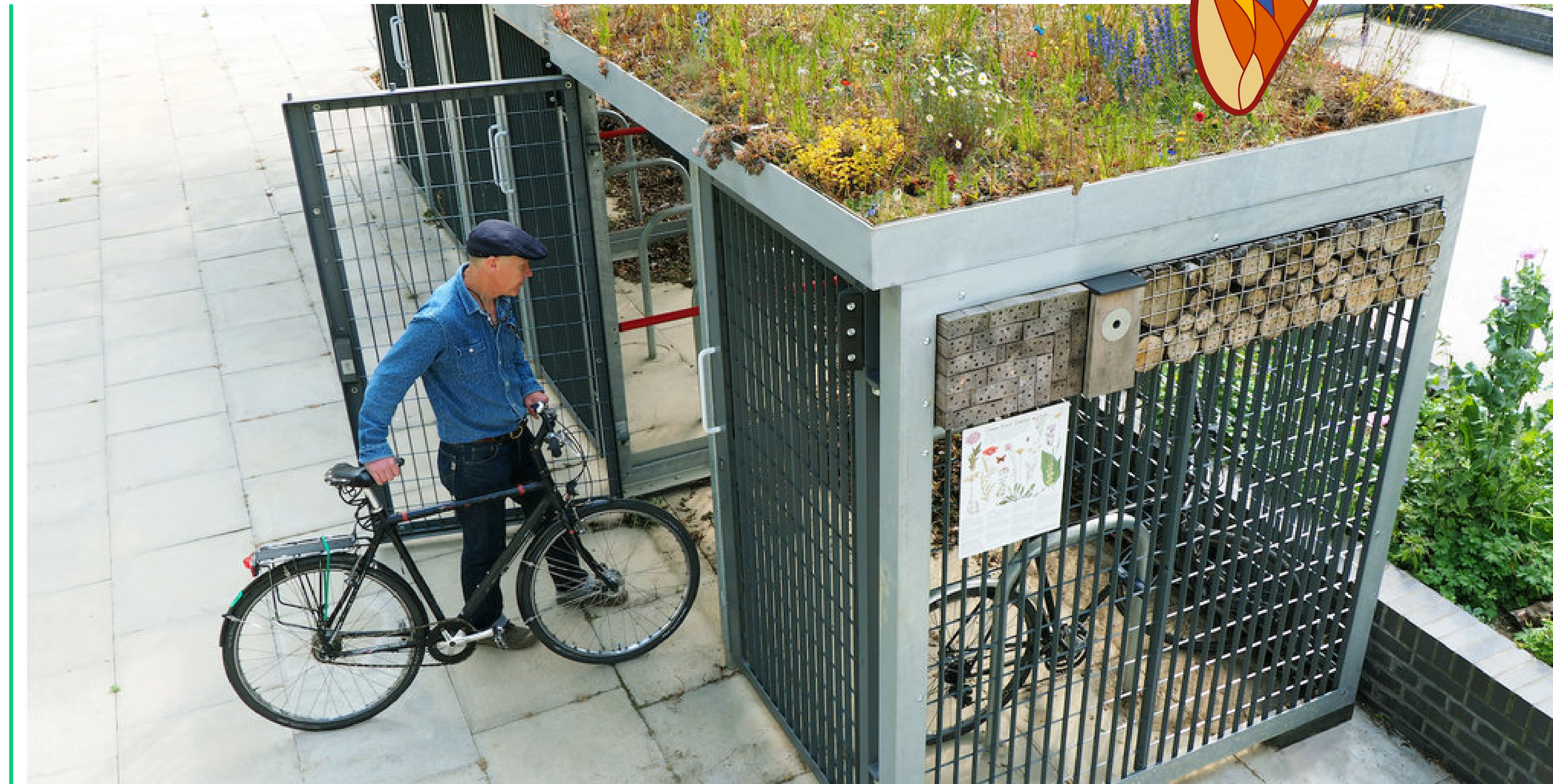
Figure 1.5 Bike shelter living roof (image credit: Green Roof Shelters)
