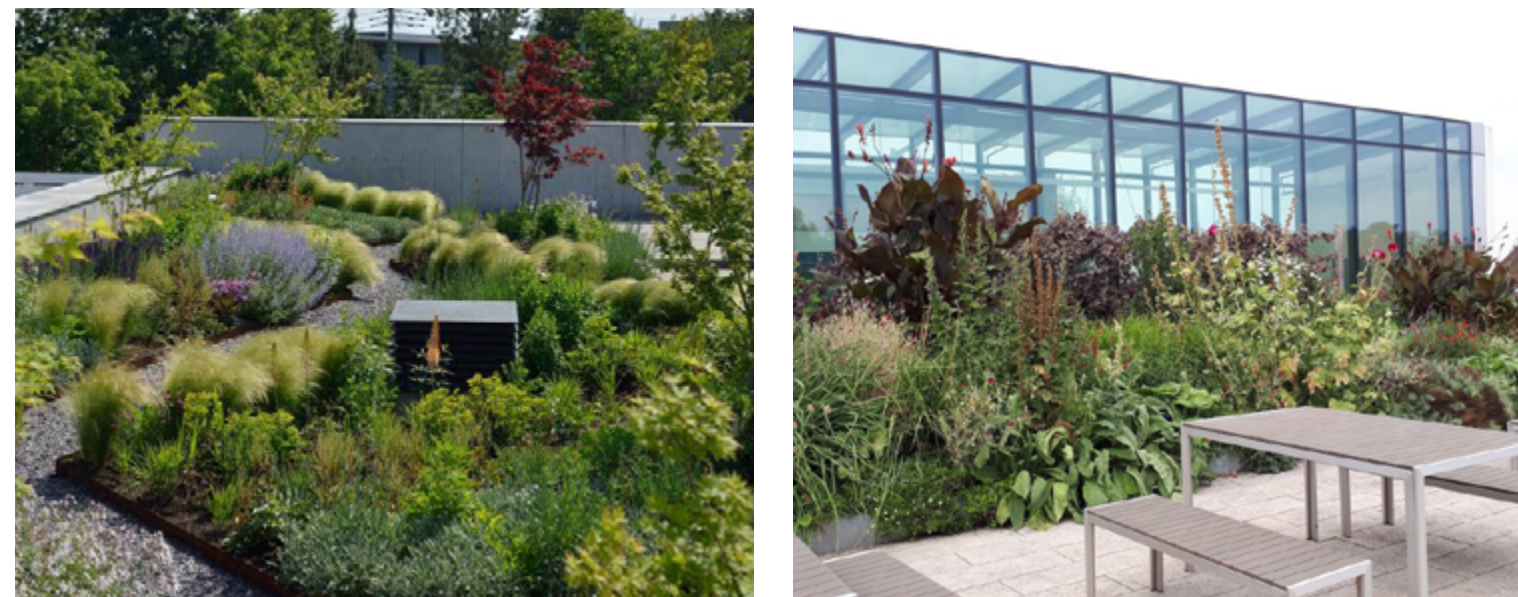
Figure 1.4 Example intensive green roofs at 20 Triton Square (image credit: Architect's Journal) and University of Greenwich which integrate amenity use with drought tolerant/biodiversity friendly design
