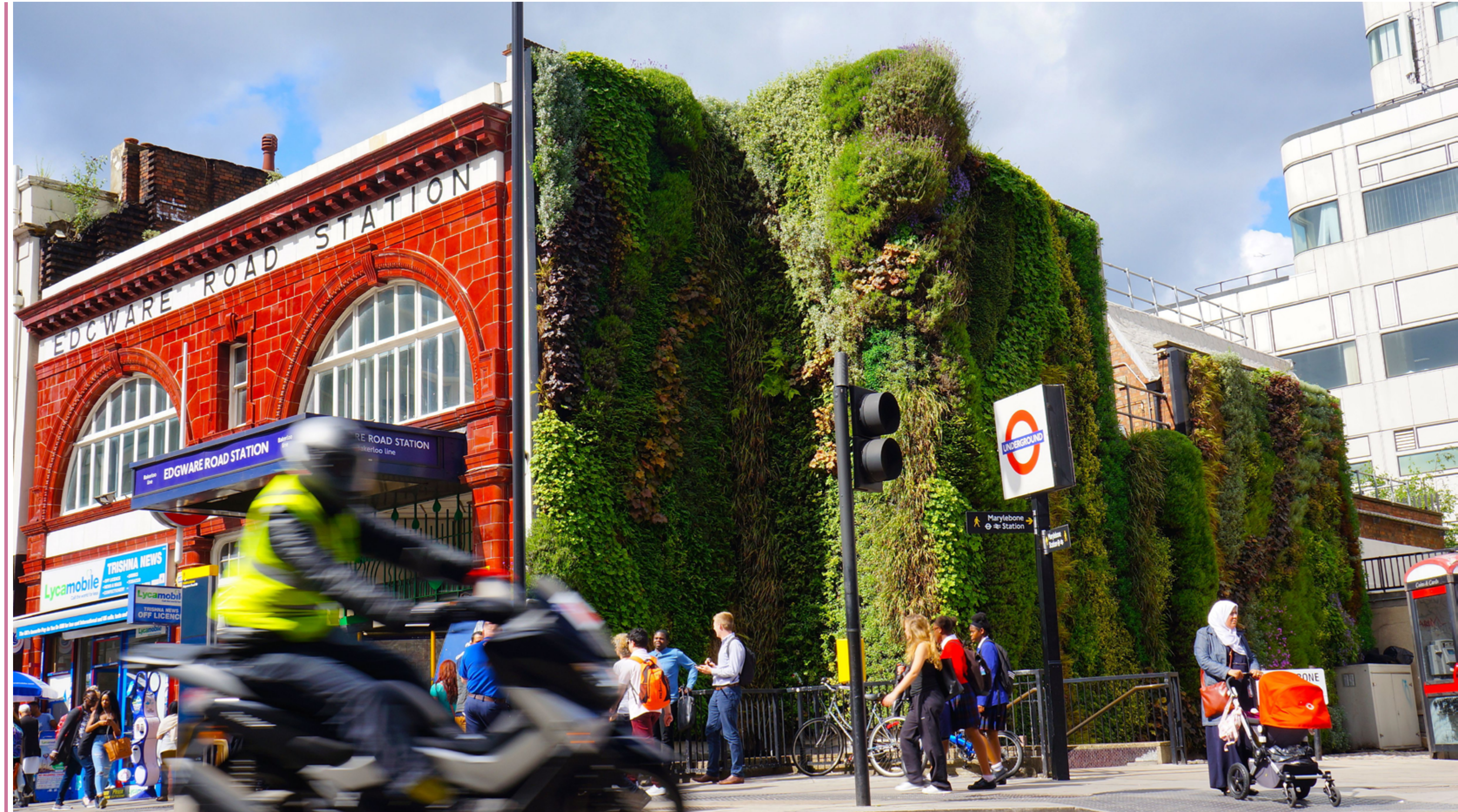
Figure 1.7 Biotecture living wall at Edgware Road station (image credit: Biotecture)
