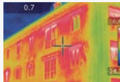
Thermal camera shots of external façades helped us to prioritise building fabric upgrades.
