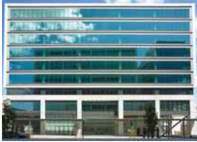
Left and above 25 Smith Street
